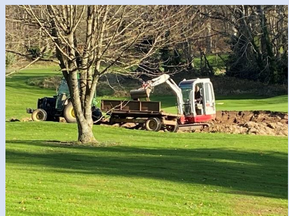
Work at the bunker at the 10 th Green
