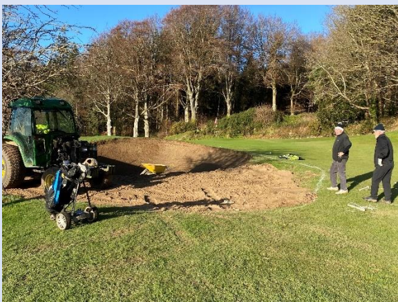
Work on the bunker at the 8 th hole
